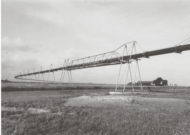
Figure 7.2 The Niederung Eden Riepe is being filled via a 13 km long pipe transporting the dredging sludge over the Ems-Jade channel (period 1946-1989). (Source: Creative Commons Attribution 4.0 International License Photo HB01395.jpg )
